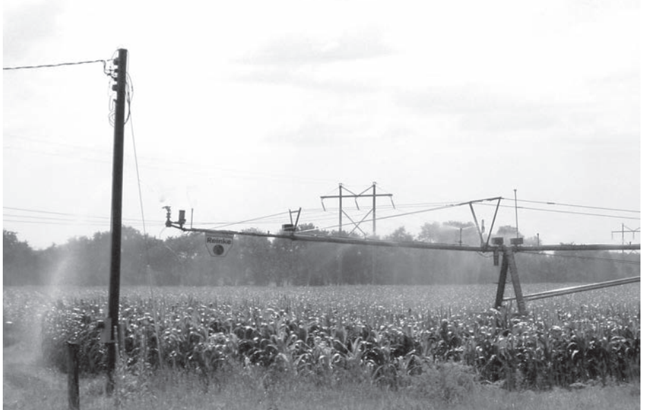
Keep irrigation equipment a safe distance from power lines.
