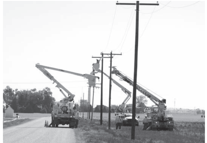
MCREA line crews rebuild existing power lines and poles. The work will continue throughout the year. (Lanett R. Schlidt, acct #xxx8400)
