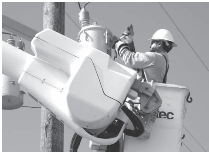
MCREA linemen work for you, our members.
