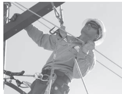
Electric lineworkers perform a variety of tasks in their job, including working on overhead lines and substations.
